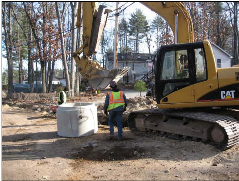
Drainage structure being placed along Shore Drive
