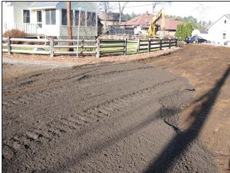
Placement of crushed gravel along Shore Drive prior to paving.
