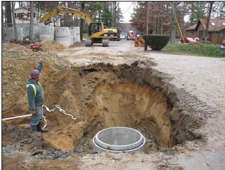
Installation of drainage structure along Shore Drive
