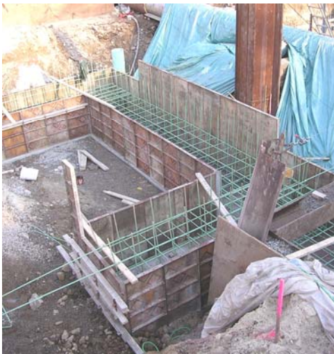
West Bridge Footing - Reinforcing steel and form work (above left) and new footing after concrete pour (above right)
