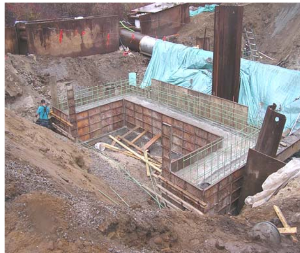
West Bridge Footing - Reinforcing steel and form work (above left) and new footing after concrete pour (above right)
