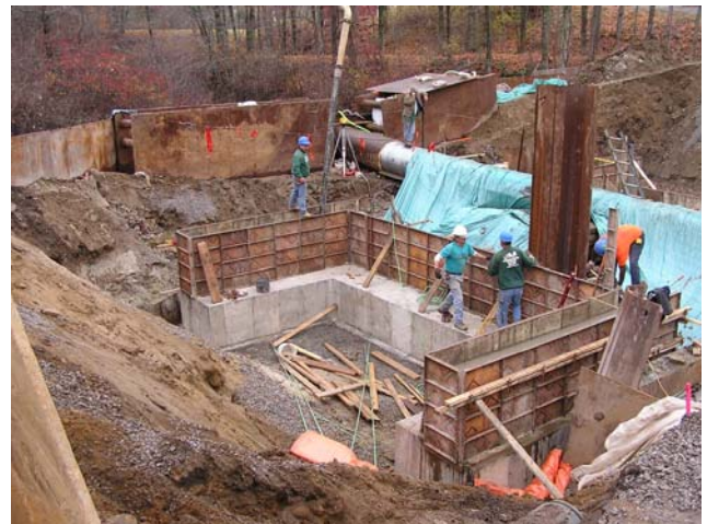
West Pedestal Wall Form work and reinforcing steel (above left) and concrete pour (above right)
