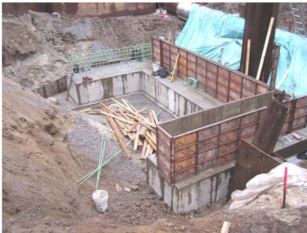
West Pedestal Wall Form work and reinforcing steel (above left) and concrete pour (above right)
